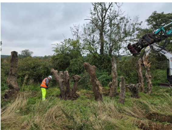
Image 12: Example monolith installation
